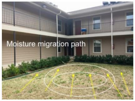
Courtyard was observed to be migrating water toward the northeast corner of the courtyard. It was not determined what the origin of this water is or at what depths. This is an area for pilot wells to determine depths and volume.
