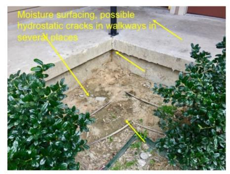
The surfacing of water in the area immediately adjacent to Unit 114 from subsurface water indicates that water migration is occurring most severely in the courtyard (NE corner). Possible hydrostatic
