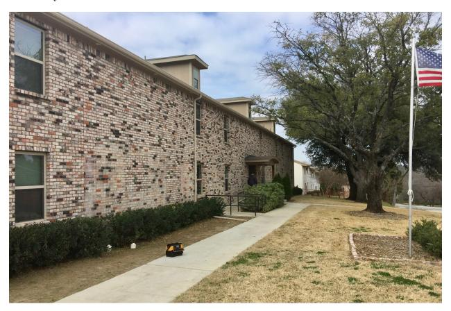
The north and west side of the property have a gently sloped yard that allows run-offs to carry heavy rain away from the structure into the local creek which is sufficient. There is a drop off approximately 28 inches on the west side of building (slope: 4.9 degrees away from structure).
