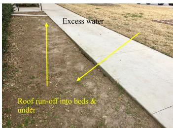
Run-off from gutter kick-outs is into the flower bed allowing more water to stand and accumulate in this area.
