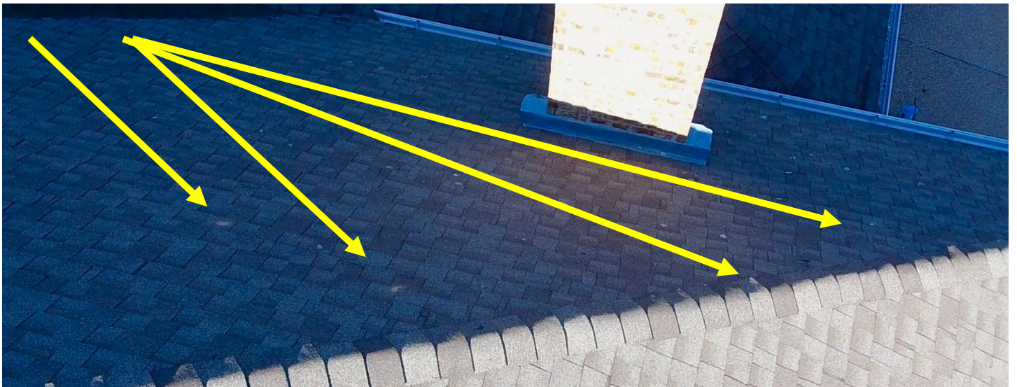
Areas of previous repairs and resealing of hail head pops
