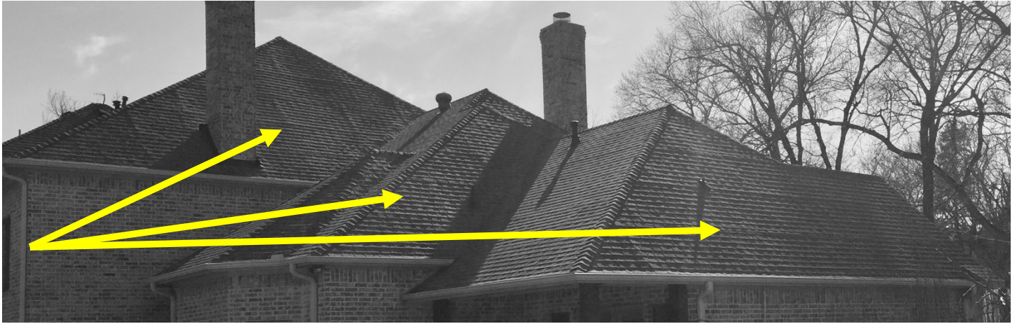
Areas of previous repairs and resealing of hail head pops
